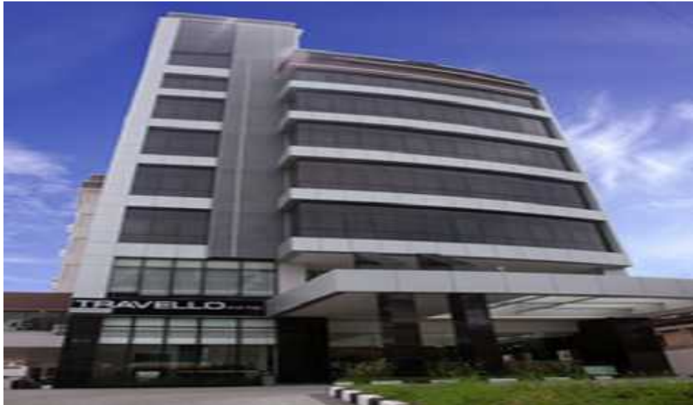
Gambar 2. Gedung Travello Hotel Manado
