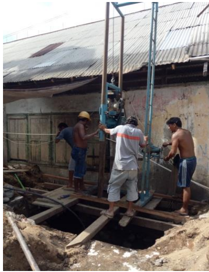
Gambar 5.32 Pengeboran Pondasi Bored Pile
