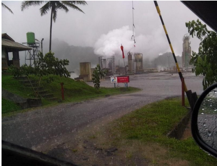
Gambar 2.3 Instalasi Pengeboran Panas Bumi PT.Pertamina Geothermal Energy (PGE) Unit 1 Cluster 13 Lahendong.
