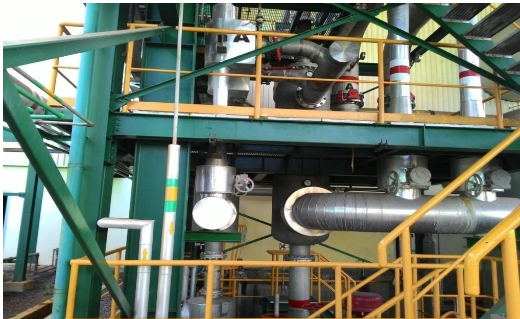
Gambar 3.9 Inter Condenser dan After Condenser
