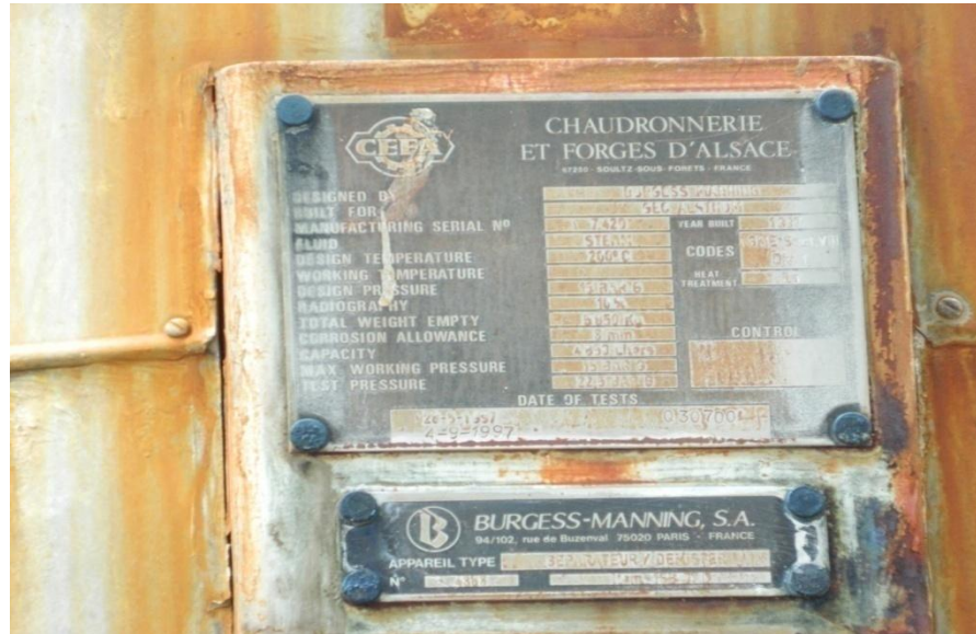
Gambar 2.7 Name Plate Demister Unit 1 PLTP lahendong
