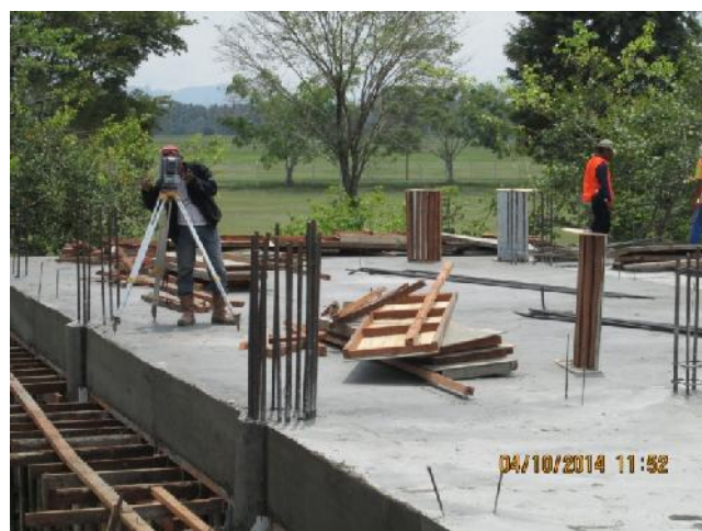
Gambar 3.61 Pengontrolan As Kolom
