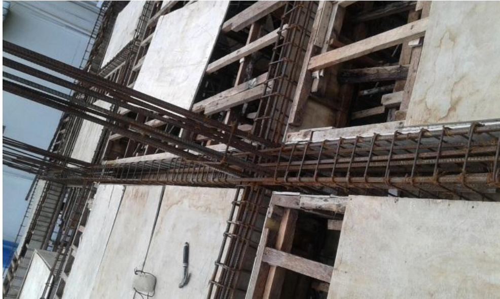
Gambar 3.12 Bekisting Balok
