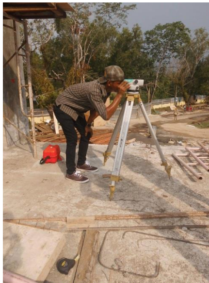
Gambar 3.28 Pengontrolan As Kolom
