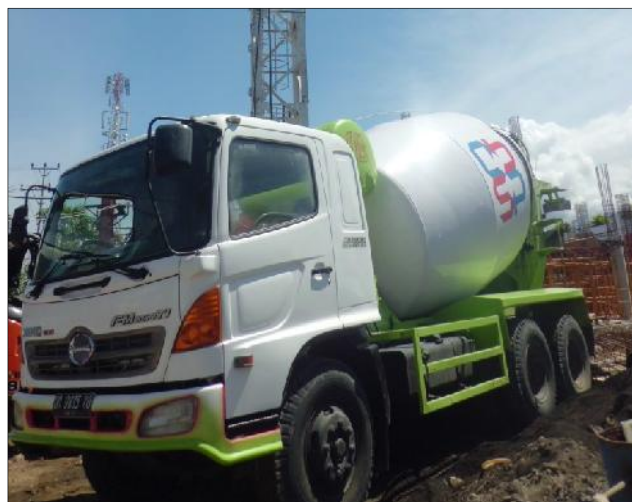
Gambar 3.32 Truck Mixer Beton Ready Mix Saat Pengecoran
