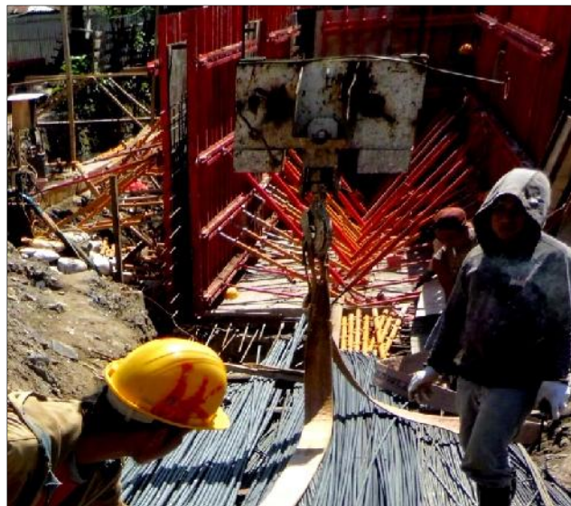
Gambar 3.31 Pelaksanaan Bekisting Propped Wall
