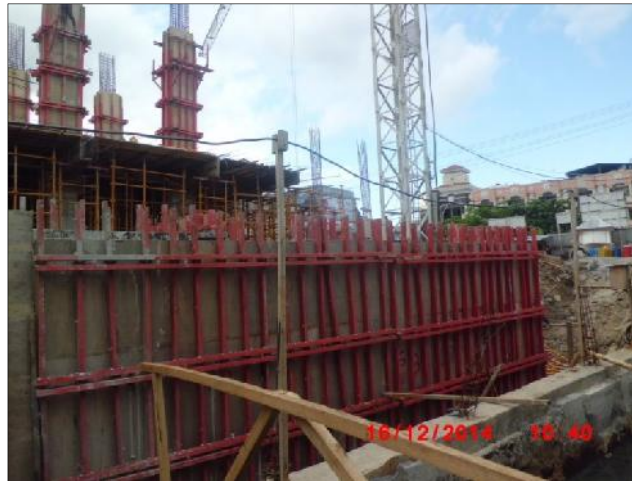
Gambar 3.30 Tampak Belakang Bekisting Propped Wall
