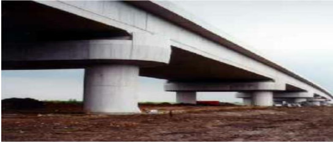
Gambar 2.6. Jembatan beton ( concrete bridge )
