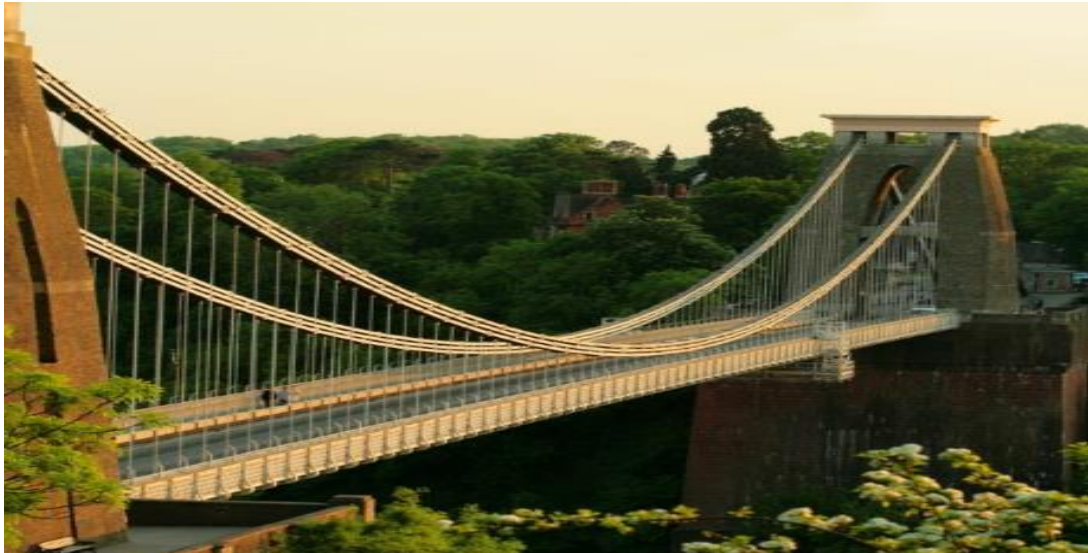
Gambar 2.4. Jembatan gantung ( suspension bridge )
