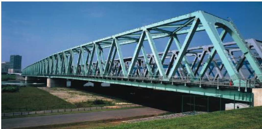
Gambar 2.3. Jembatan rangka ( truss bridge )
