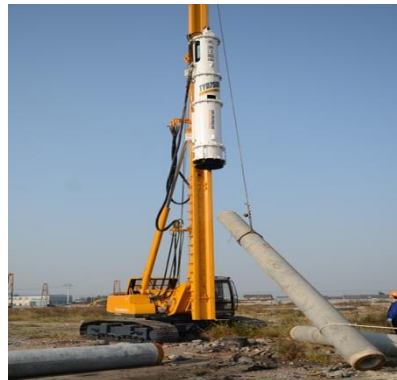
Gambar 2.10 Drop Hammer
