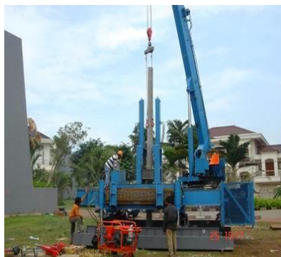
Gambar 2.12 Hydraulic static pile driver
