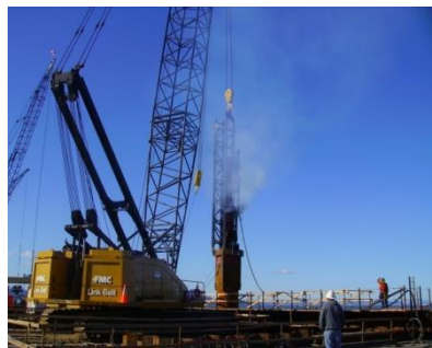
Gambar 2.11 Diesel Hammer
