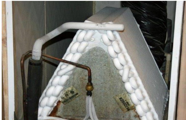
Gambar 9. Evaporator AC
