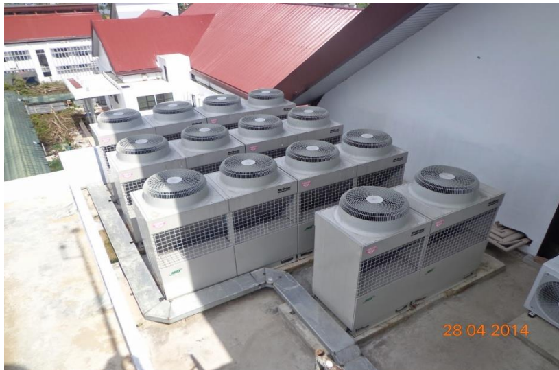
Gambar 5. AC Central Unit Outdoor(Luar)
