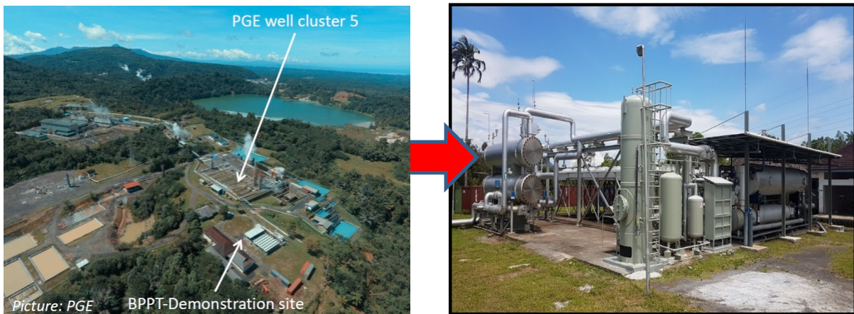
Gambar 1. Lokasi Lahendong Pilot Plant Binary Cycle 500 kW
