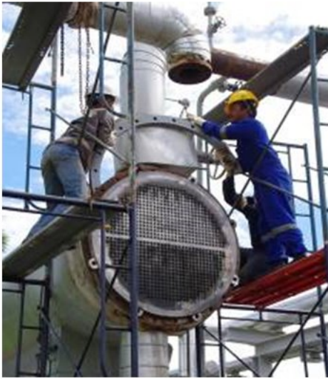
Gambar 4. Proses maintenance flange heat exchanger
