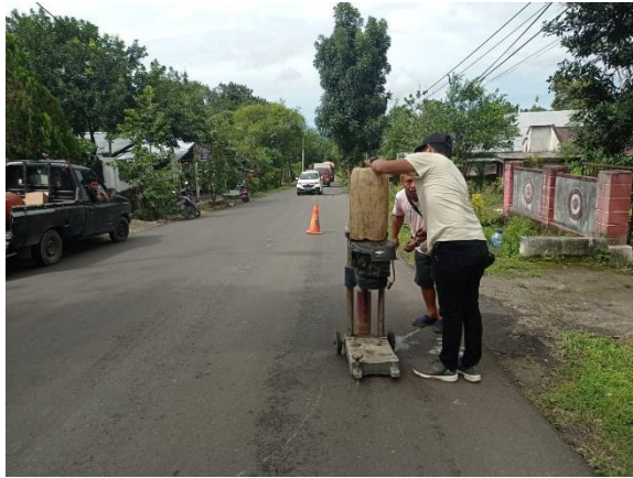
Gambar 3.3.5 Pengambilan Sampel Core Drill
