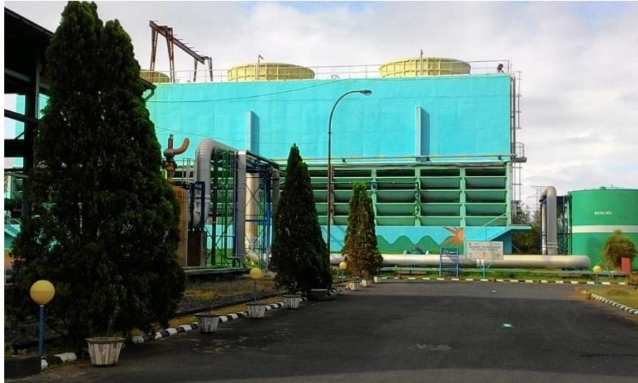
Gambar II.4. Menara pendingin ( cooling tower ).
