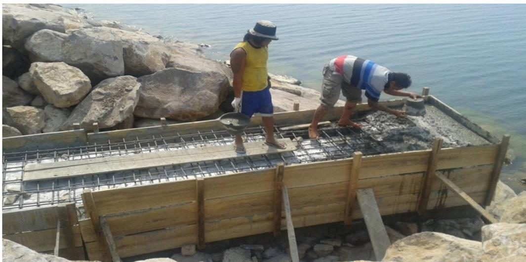
Gambar Pengecoran Cross Drain
