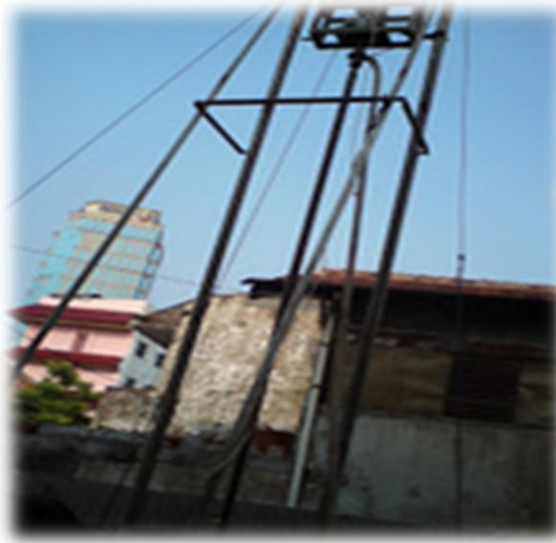
Gambar 2.9 Bored pile gawangan
