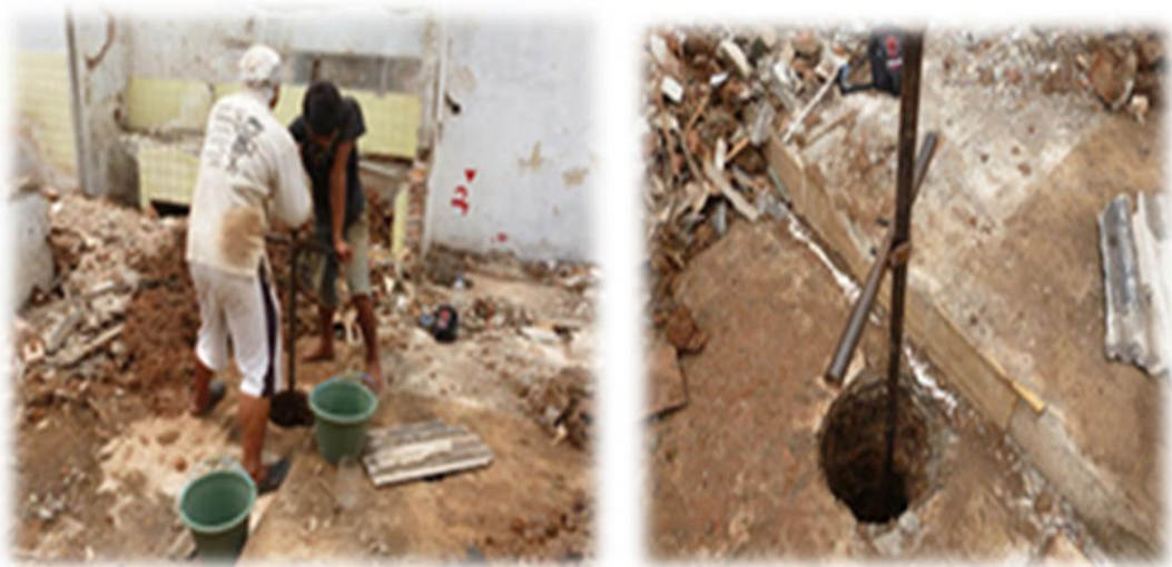
Gambar 2.10 Bored pile manual
